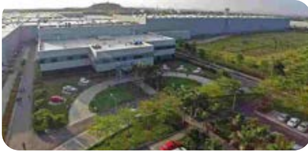
Two stage evaporative cooling with capacity- 1100000CFM for body shop, engine shop, PT shed and CVA.
