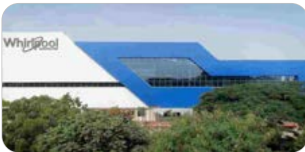
Whirlpool India Ltd, Ranjangaon- 1500000 CFM single stage evaporative cooling.
