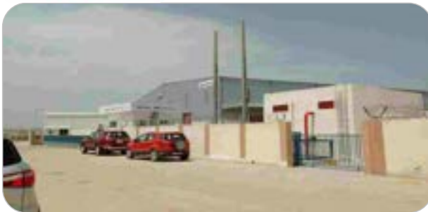
Getrag Transmission India Pvt Ltd, Sanand- 240000 CFM two stage evaporative cooling.
